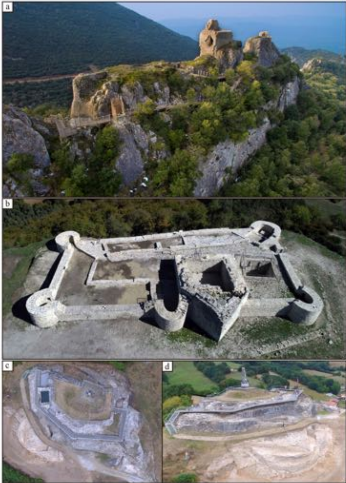
Figure 2. Historical buildings to which the studied lime mortar samples belong. (a) Portilla Castle. (b) Irulegi Castle. (c, d) Amaiur Castle.
