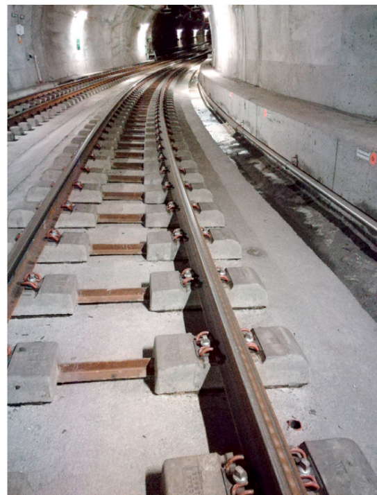
Fig. 2. Corrugation found in the line under study.
