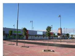
Parking permeable adoquines. Madrid
