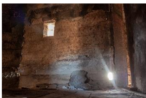
Figure 1. Fresco fragments detached from the wooden beams of the Amărăști church
