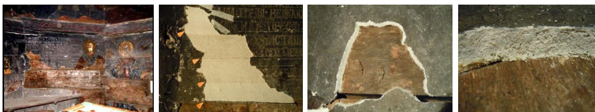
Figure 1. In situ application of the restoration mortars
