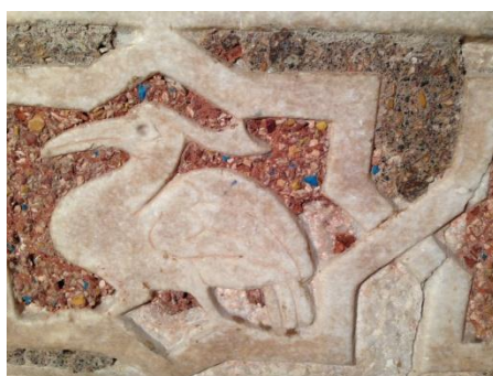
Figure 1. Marble panel with mastic incrustations – Presbytery, San Nicola Church (Bari, Italy)
