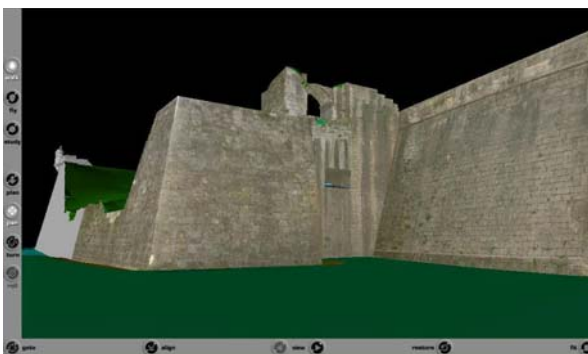
Fig 5: In the first picture the building can be seen in parts, selecting them in the right menu. In the second one, a hierarchically organized model is shown, the parts of the model that are closer to the viewer appear with photographic rendering and the other ones with colour rendering.
