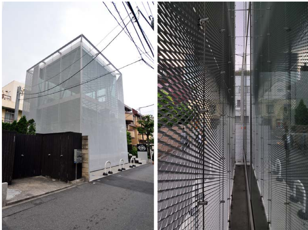
Fig. 2.7. Carina store. Tokyo 2012. SANAA architects 2009. https://www.flickr.com/photos/kirabelle9/ https://creativecommons.org/licenses/by-nc-nd/2.0/
