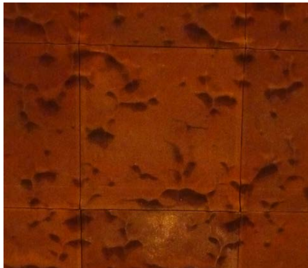
Fig. 2.28. Embossed EM mesh cladding. Caixa Forum basement auditorium. 2011. Herzog&deMeuron architects. Manufacturer: IMAR.
