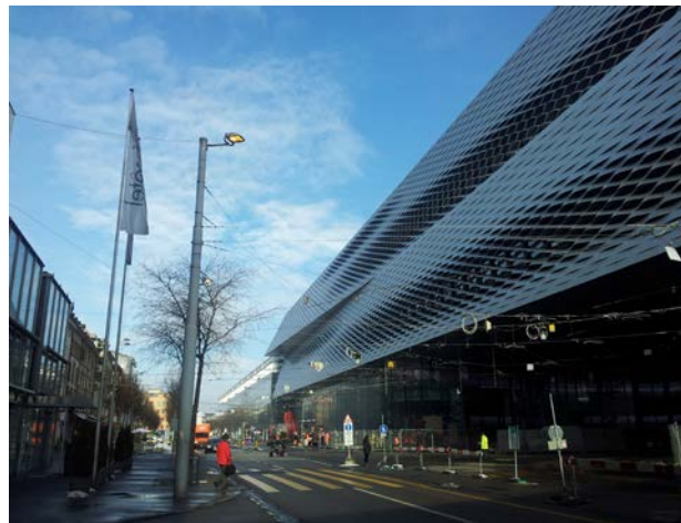
Fig. 2.24. Messe Basel. Exhibition Hall. 2013. Architects: Herzog & de Meuron. https://www.flickr.com/photos/patsch/ https://creativecommons.org/licenses/by/2.0/
