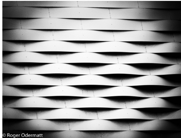
Fig. 2.26. Messe Basel. Exhibition Hall. 2014. Architects: Herzog & de Meuron. https://www.flickr.com/photos/rogerodermatt/ https://creativecommons.org/licenses/by-nc-nd/2.0/
