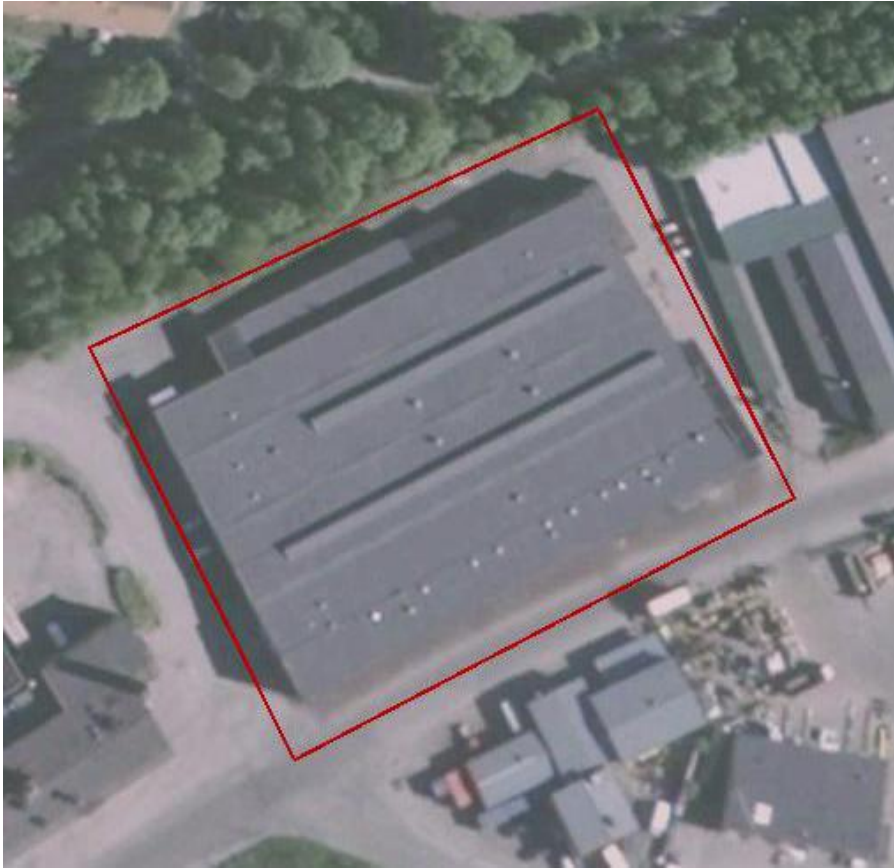
Figure 4: Satellite view of the roof of the building. Source: Google Earth
