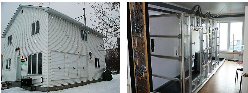
Figura 1.14 – FEWF, Field Exposure Wall Facility, del NRC-IRC de Canada
