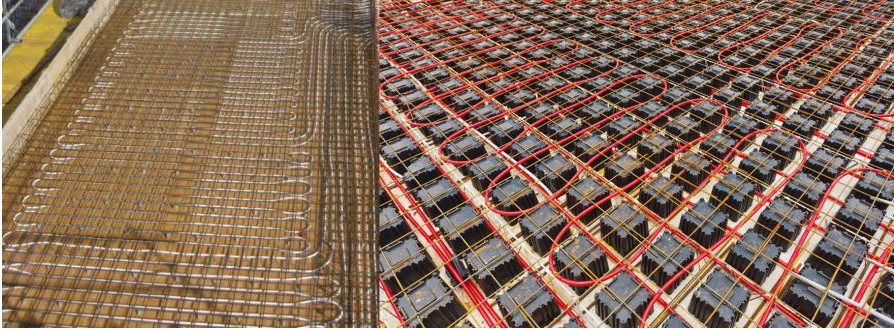
Figure 3.5. Water pipe preparation before dropping the concrete to create TABS slab
