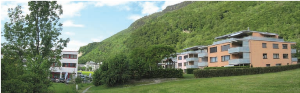
Fig. 9: This group of residential buildings makes use of the potential of the landscape structure formed by the former outer bank of the Rhine; Triesen. (Catarina Proidl)
