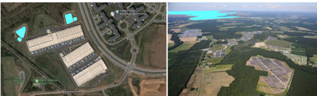
Fig. 7. Presente y Futuro de los centros de datos de Amazon AWS. AWS data center in Northern Virginia and Amazon Solar Farm Virginia, 100mw. Present and Future of Amazon AWS Data Centers. AWS data center in Northern Virginia and Amazon Solar Farm Virginia, 100mw ( https://www.google.es/maps ).
