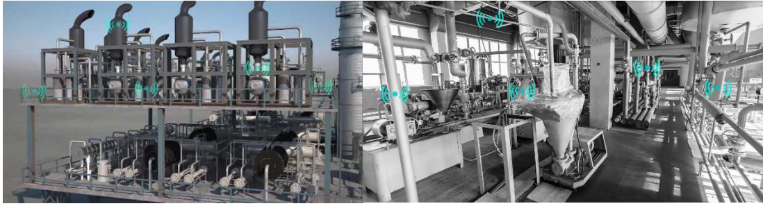
Figure 1-10: Examples of IIoT application in a refinery industry.
