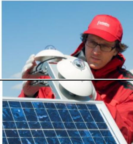
Figure 2 PV system performance monitoring pyranometers
