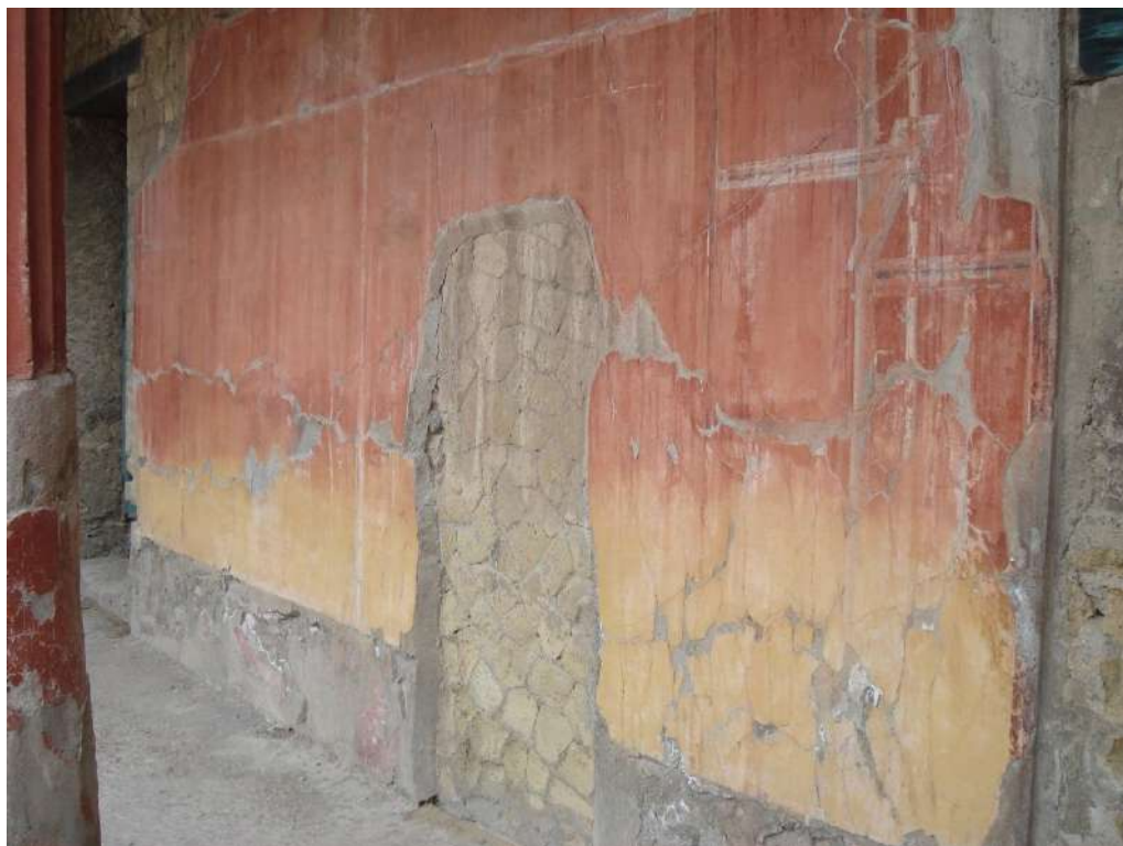
Fig 2. Wall painting from Pompeii showing the transformation of yellow ochre into red in its middle-upper part.
