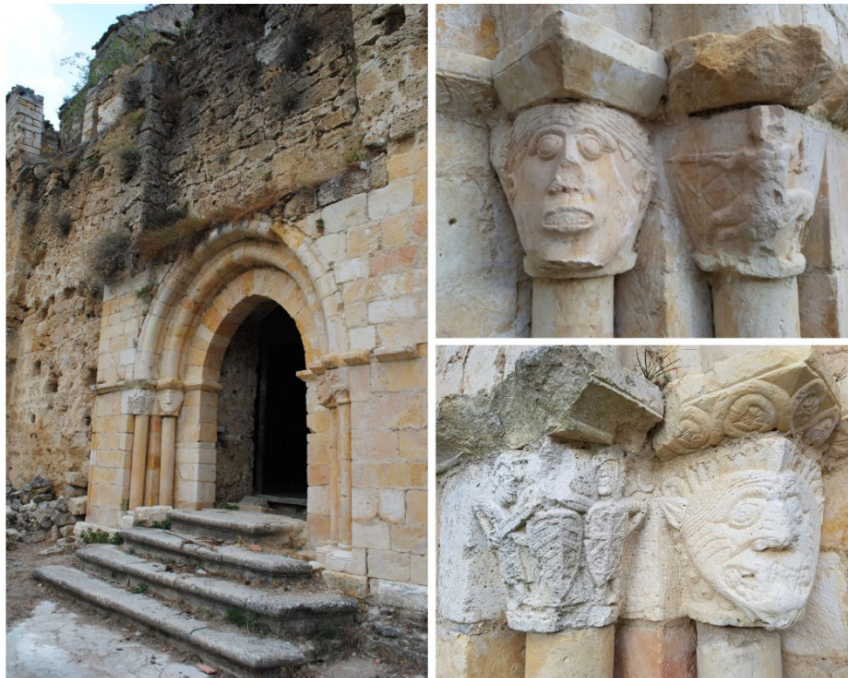
Figure 3.3: Romanic portal and particular of carved capitals.
