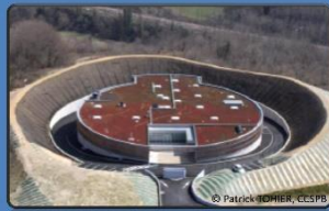
Fig.1: Water Treatment Plant (WTP)
