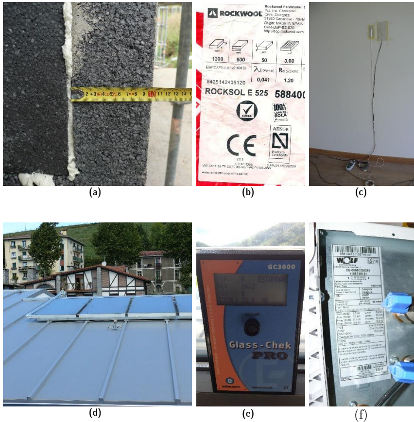
Figure 3.2. In-situ visual inspections and measurements: (a) measurement of insulation thickness; (b) insulation label collected in building works; (c) in-situ thermal resistance test; (d) solar thermal collectors verification; (e) window glass thickness and low emissivity measurement; and (f) boiler label verification.
