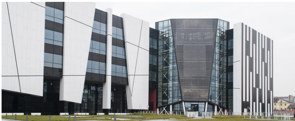
Figure 1. Energy Center from the outside.
