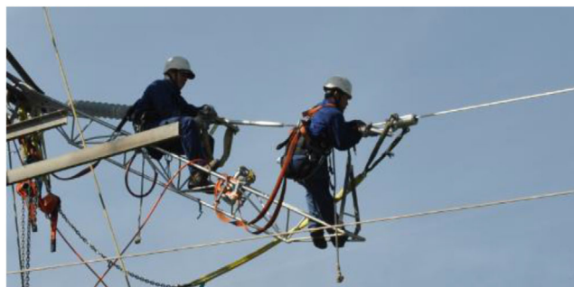
FIGURE 2 Installation of the GTACSR conductor
