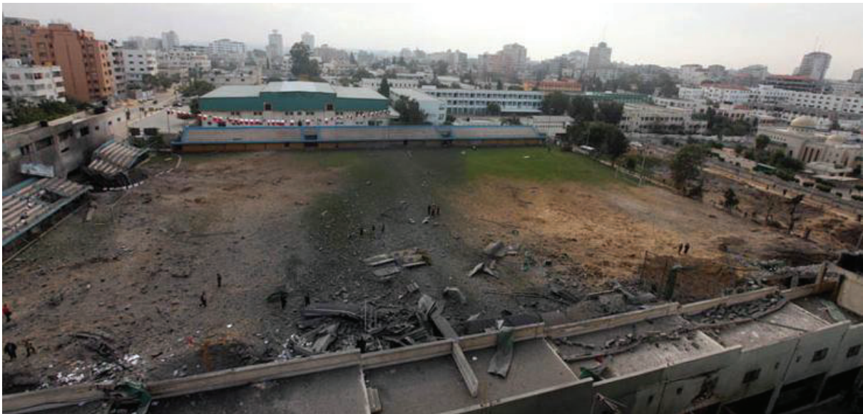
Figure 13 Palestine stadium in Gaza after being bombed by the Israeli army
