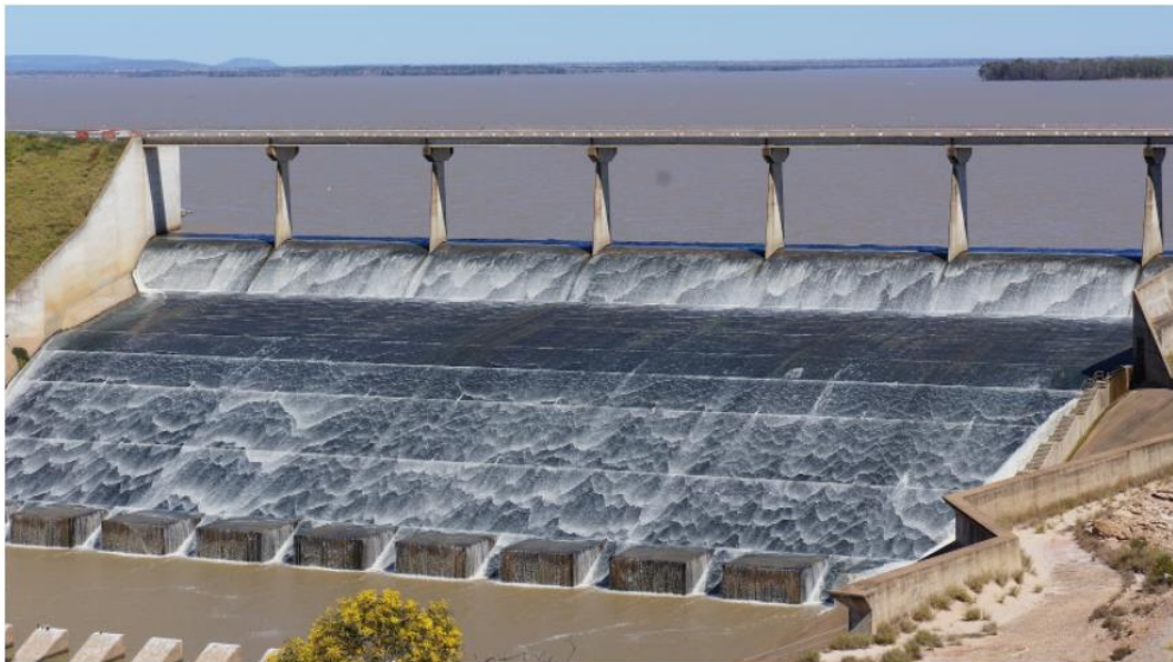
Figure 1-Ogee crest spillway example
