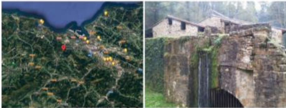
Figure 31 – On the left, location of the “El Pobal” ironwork. On the right, the ironwork
