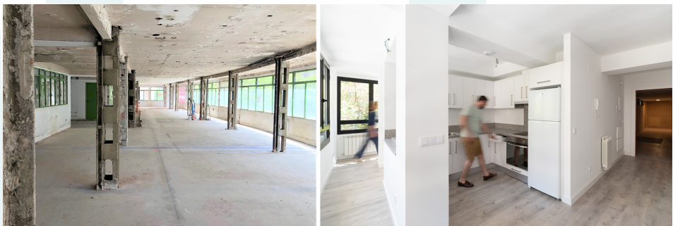
Figure 8. Structure and internal ceilings a) Photo Geo2, 2020. B) Photo Ana Matos 2022
