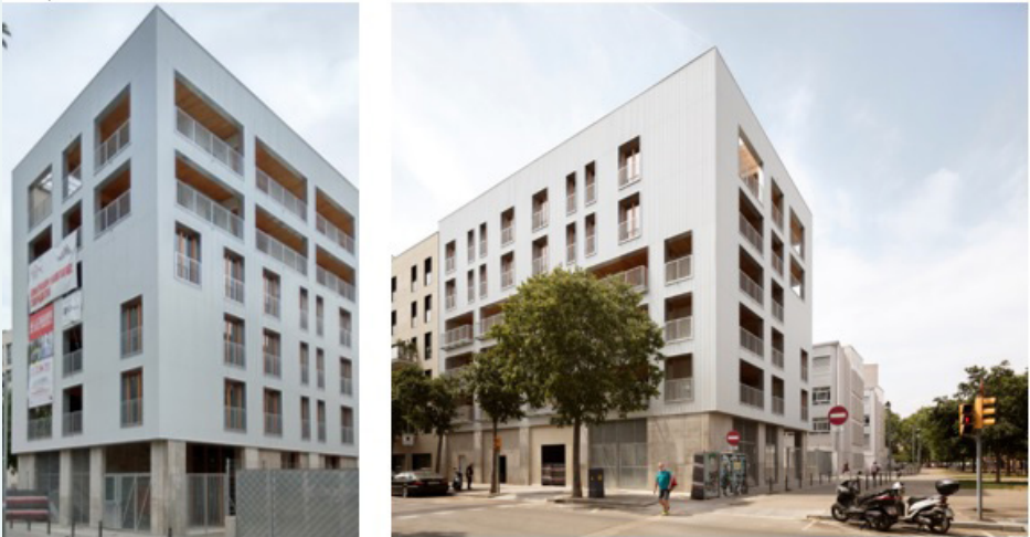
Figure 1. La Balma exterior view [4]
