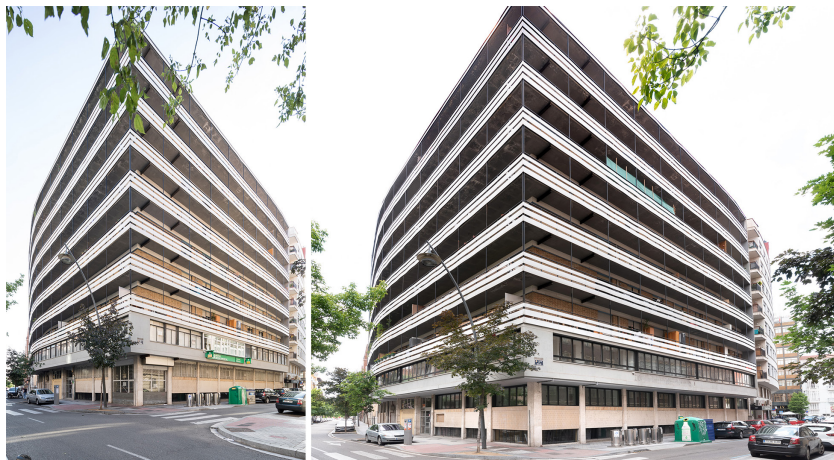
Figure 1. Intervention c/ Muro 16, before / after. a) Before. Photo. P. Iván, 2018. b) After. Photo Ana Matos. 2022
