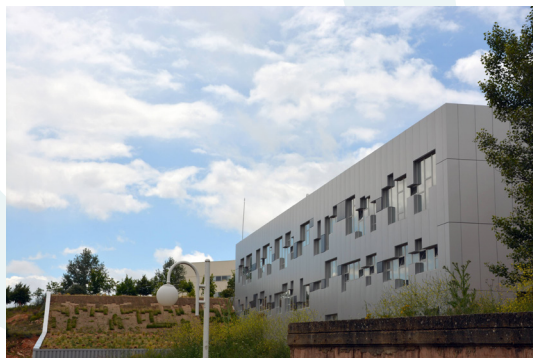
Figure 4. The semi-buried Southwest facade connects with the corridor area, and facilitates views, natural ventilation and also houses the facade with vertical photovoltaic panels. 10
