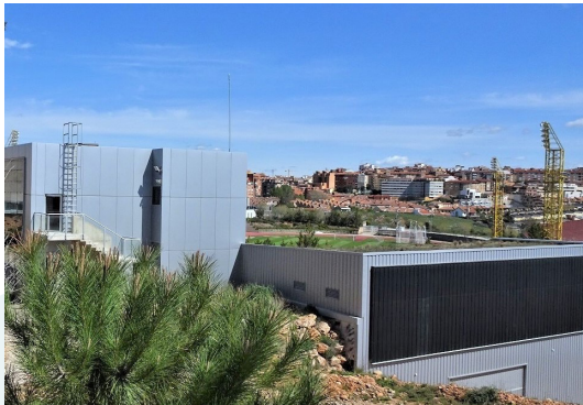
Figure 3. Solar wall for air preheating, and green roof . Photo: MJGD.2021
