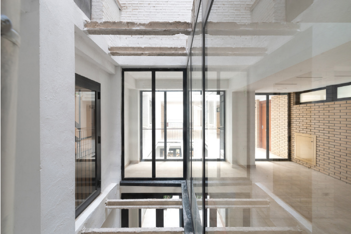
Figure 5. Extended courtyards , galleries and construcción materials. Photo: Ana Matos. 2022.
