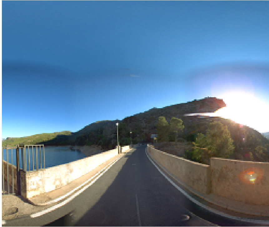
Figure 2.1: Shadows in the road due to sun position
