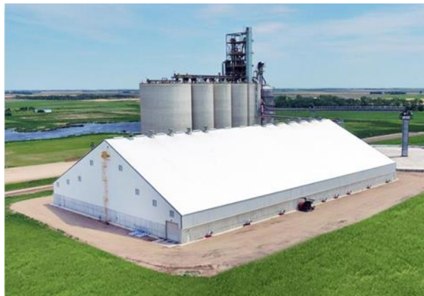
Figure 2 Flat storage system in Verona, North Dakota [2]
