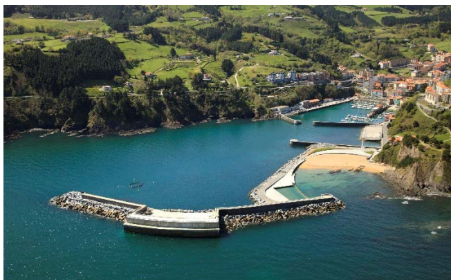
Fig. 1. Top view of the Mutriku wave power plant and the breakwater.
