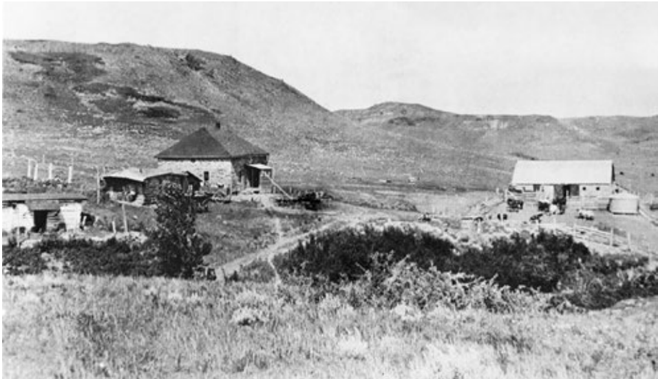
FIGURE 5 • John Etchart's home ranch—the so-called Stone House—at the head of Willow Creek in south Valley County (Montana), ca. 1920
