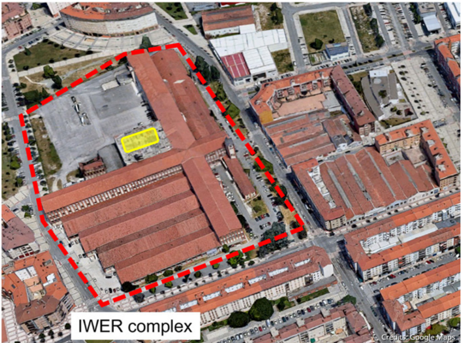
Fig.1: Aerial view of IWER complex and it's cistern.
