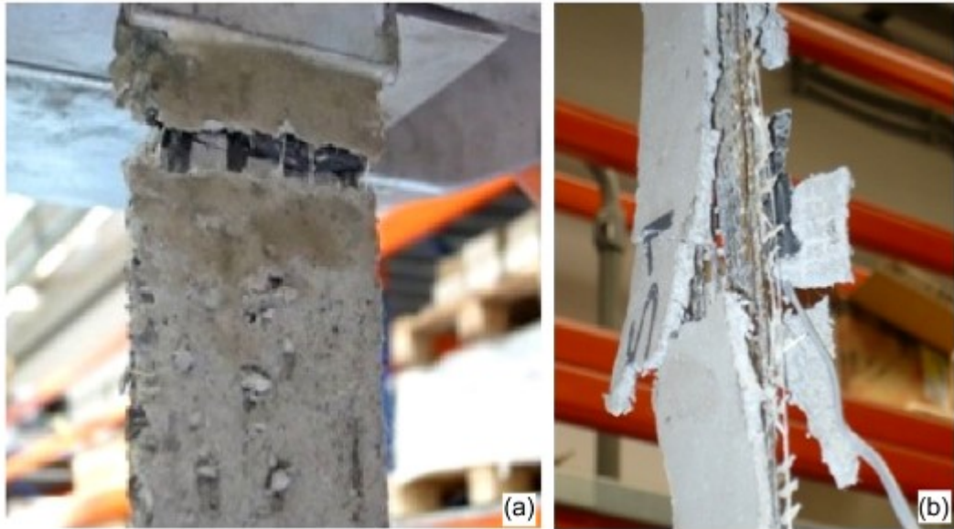
Fig. 5 Damage pattern in tensile tests: development of cracks in the vicinity of the aluminium plates in CTRM (a) and detachment of the mortar in SRG (b)
