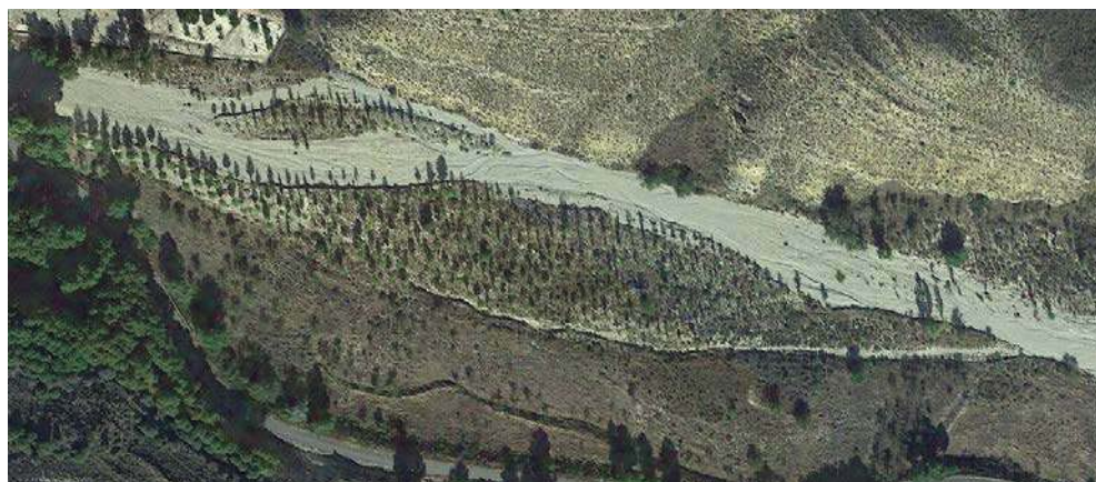
Figure 114. Planting within the channel of the Barranco de La Nava (Aguilar de Río Alhama, La Rioja)
