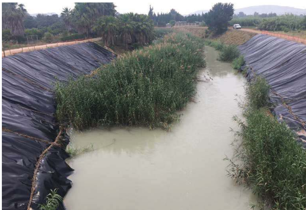
Figure 115. Example in a permanent river (River Segura in Molina de Segura, Murcia) of treatment for the elimination of reeds on both channel banks.
