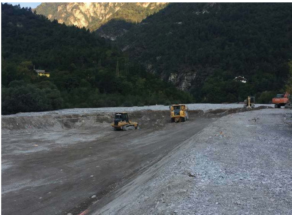
Figure 107. Bed gravel extraction in the Desedan Torrente (Longarone, Italy)
