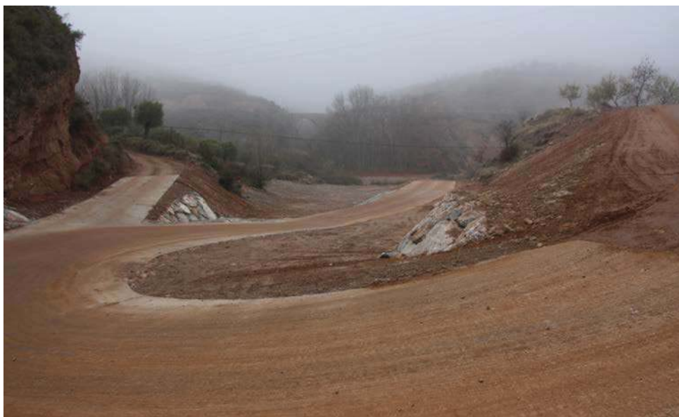
Figure 104. Tracks that have a barrier effect and invade the channel in the Barranco de la Mata (Jubera, La Rioja)
