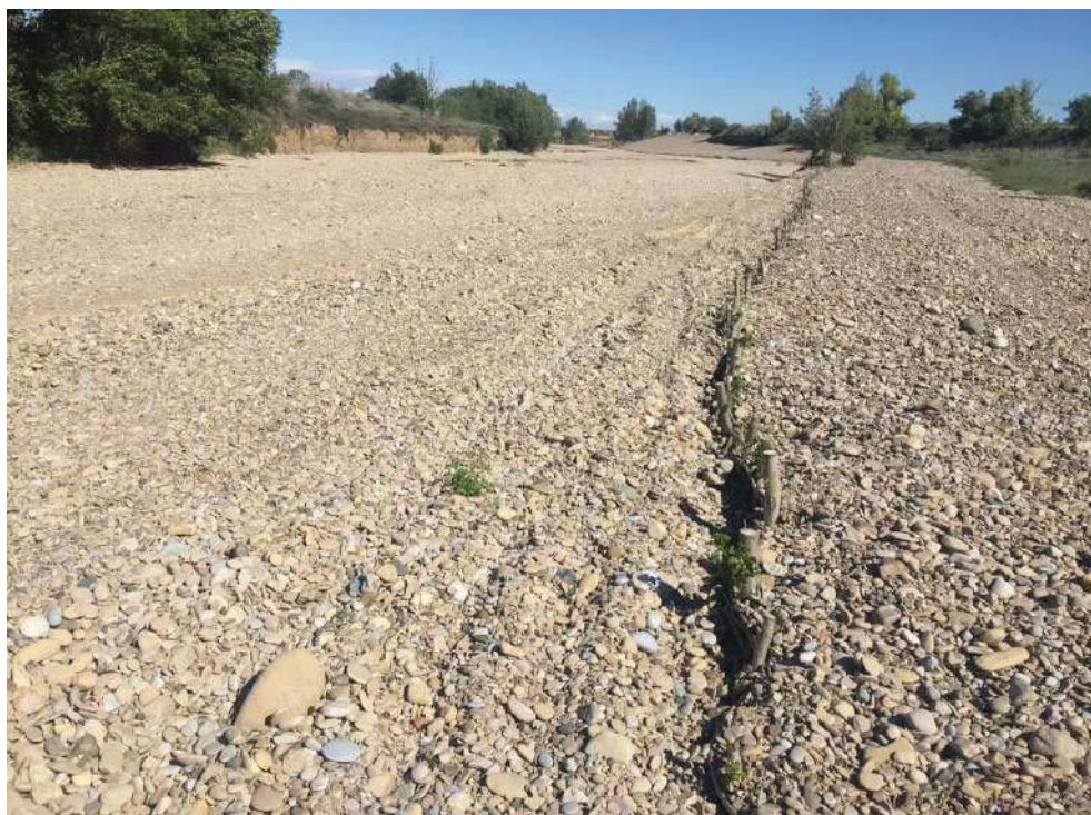
Figure 119. Bad practice of revegetation in a dry channel reach of the Arba de Luesia (Rivas, Zaragoza) altered by recovery work of the drainage cross-section. The aligned stakes narrow the channel.
