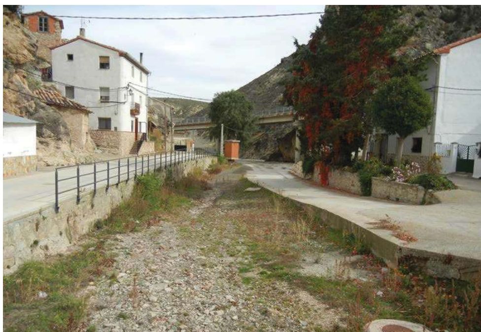
Figure 111. Pipes and collectors lead to a further narrowing of the Río Seco channel (Hoz de la Vieja, Teruel)
