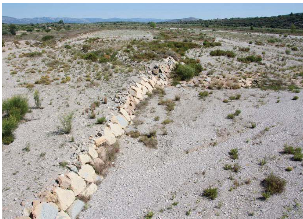
Figure 122. The Rambla Cervera (Sant Mateu, Castelló), with internal protective ripraps that cut through and restrict the channel active space.
