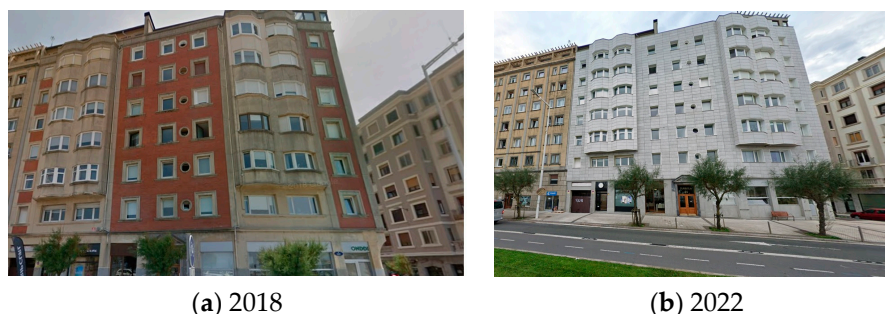
Figure 1. (a) View of a post-war building's facade in 2018, with facade of continuous render and facing brick; (b) 2022 view of the same building, renovated—the frontage has been covered with a ventilated facade, causing an evident distortion of the whole.
