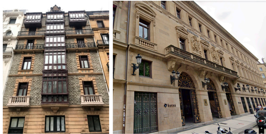
Figure 7. Unprotected eclectic buildings.
