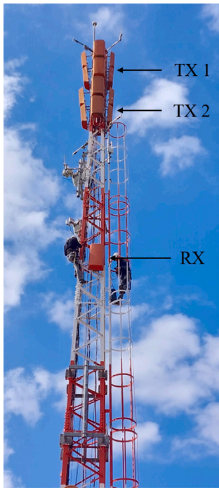
Fig. 4. The ongoing broadcast transmission tower during the measurement campaign. The transmission radiating system (TX 1 and TX 2) and the portable receiver (RX) are identified.
