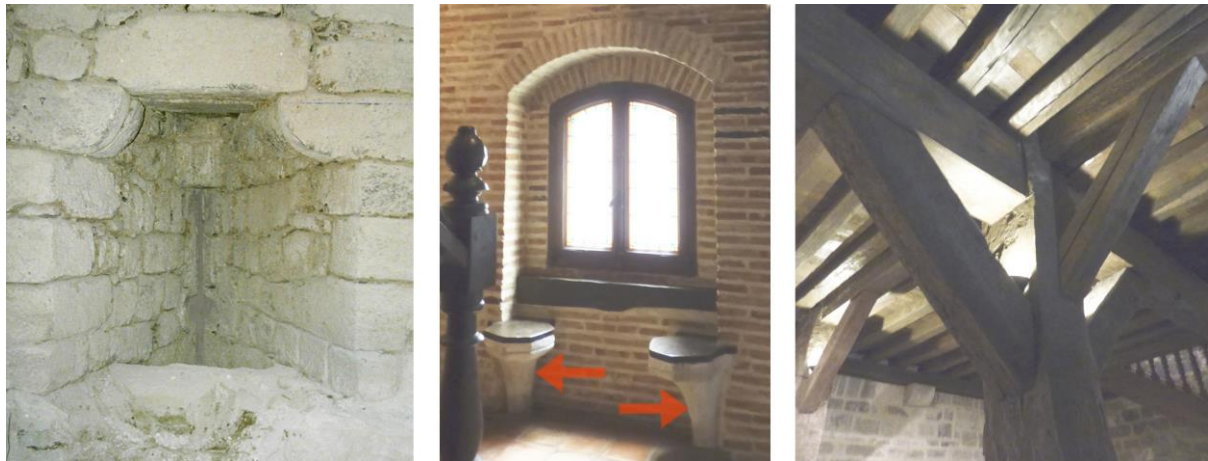
Fig. 12. Left: Inner space of the embrasure. Center: Window with original seats on the main floor. Right: Joints with strut braces in two directions. Photos: Daniel Luengas-Carreño
