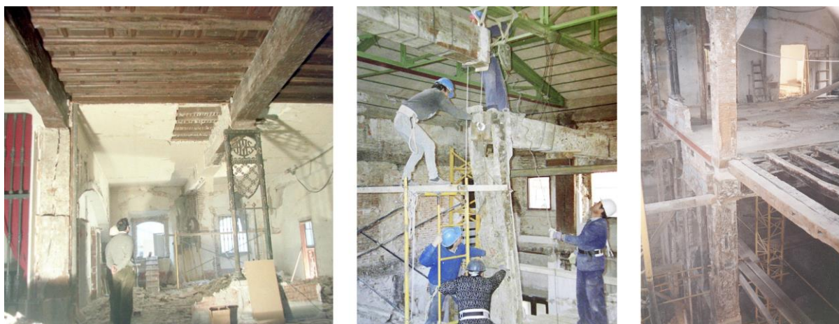
Fig. 10. Gutting of the interior of the Tower Palace. Photos: Antón López de Aberasturi
