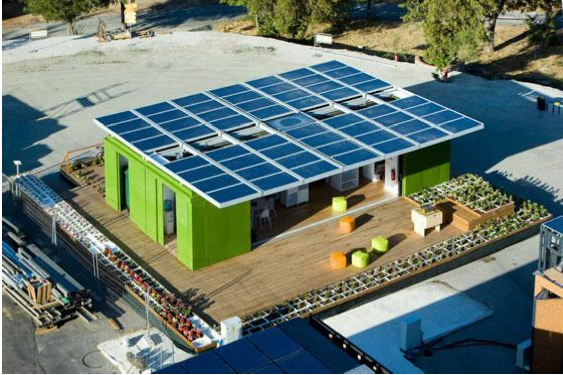
Figure 13: PV Roof of Ekihouse
