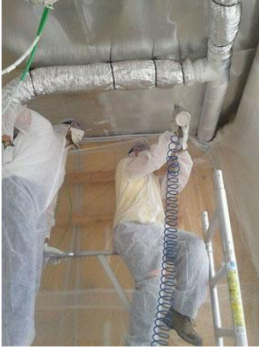
Figure 7: Installation of PCM panels in the ceiling.
