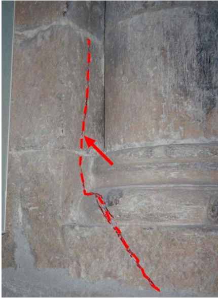
Figure 6. Some cracks in the top part and in the bottom part of a pier in the Colegiata Church in Toro city (Spain).
