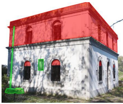
(a) Outside view of the lighthouse
