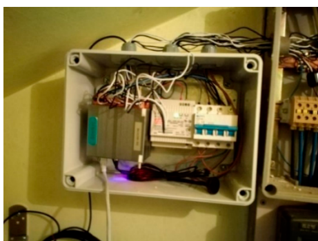
Figure 5. Installation of the datalogger (Source: Ekitermik Efizientzia Energetikoa).
