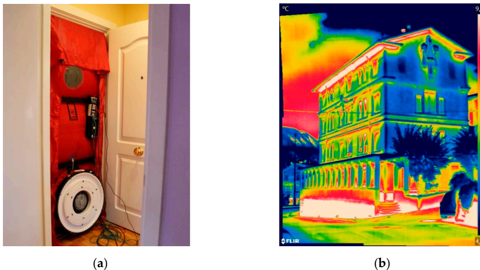
Figure 4. (a) Installation of the fan to test the permeability of the windows; (b) Thermography of the main facade. (Source: LCCE).
