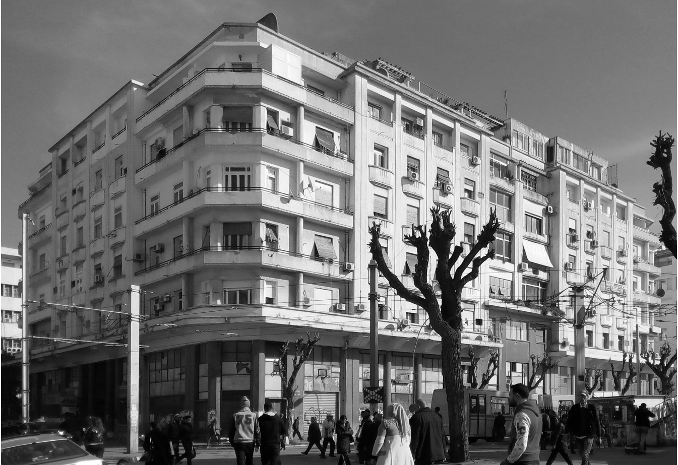
Figure 15. View of the Schwich et Baizeau block, 1936, by Joseph Hiriart and Jean-Marcel Seignouret, from the railway station square, demonstrating the imposing presence demanded by the two associates in the construction of the headquarters of the company, photographed by the author, 2019
