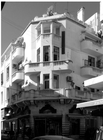
Figure 13. View of the apartment block of the Compagnie des Assurances Générales, 1934, by Joseph Hiriart and Jean-Marcel Seignouret, showing polygonal bay windows starting from the balcony of the first floor and becoming a loggia on the third floor, photographed by the author, 2019
