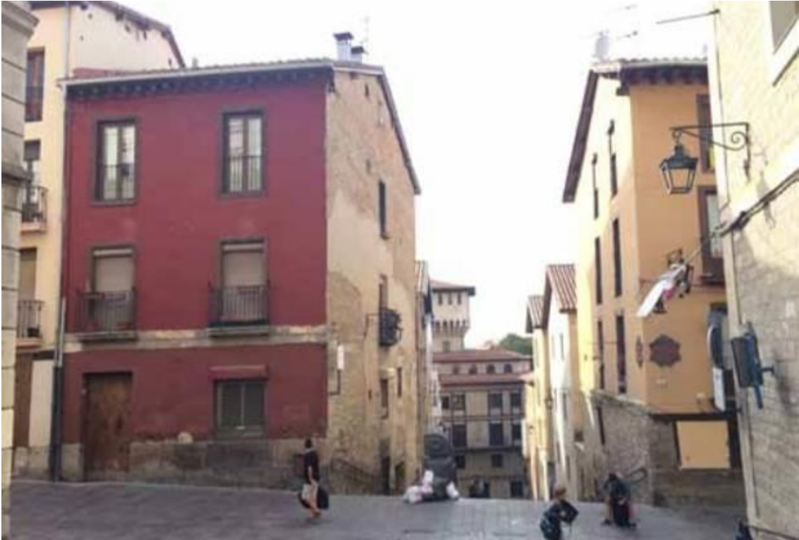
Figure A.6 - General view of the building before refurbishment
