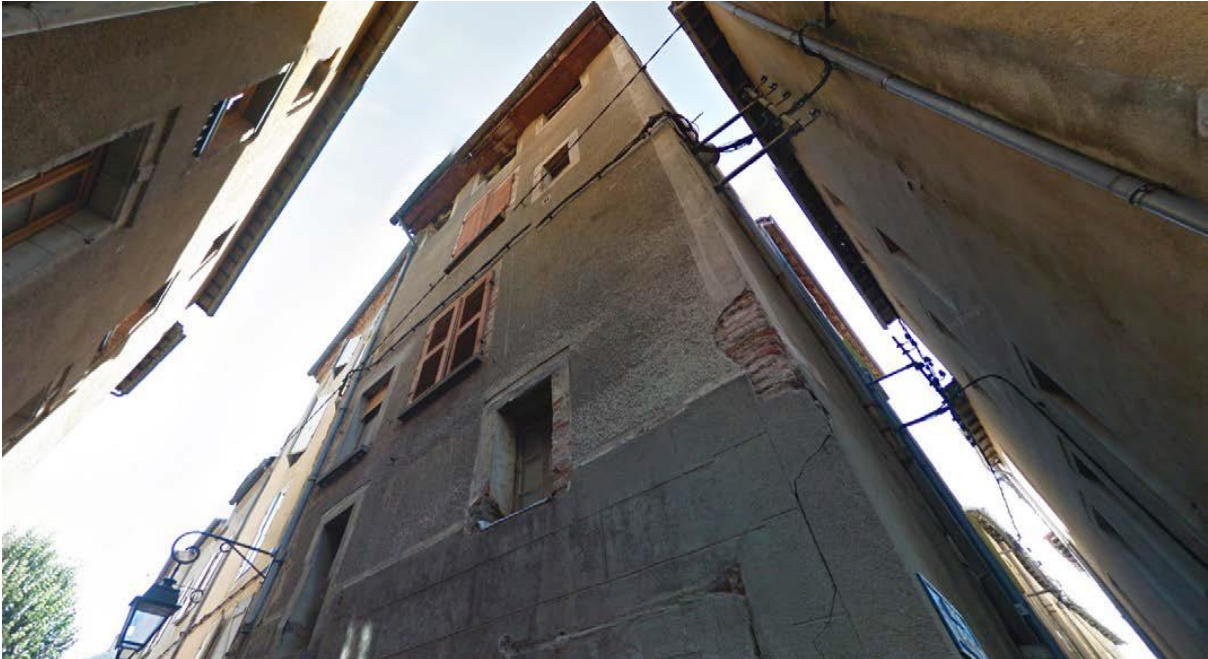
Figure A.1 – General view of the building before refurbishment
