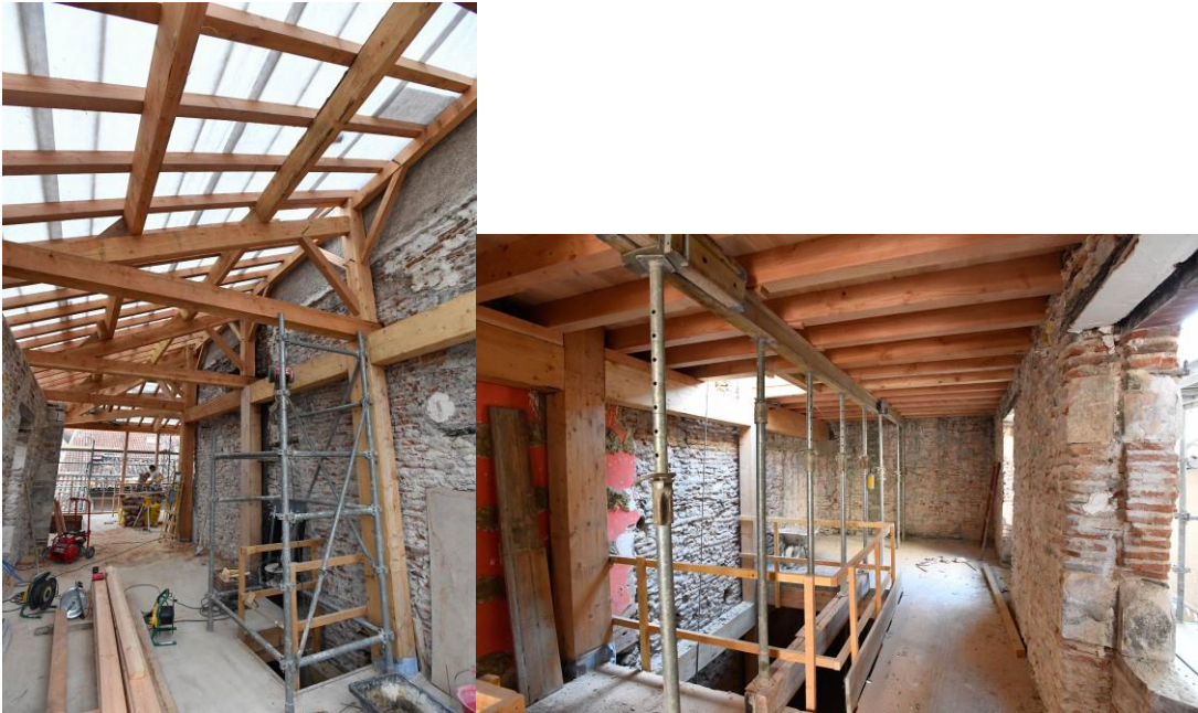
Figure A.2 - View of the building during refurbishment
