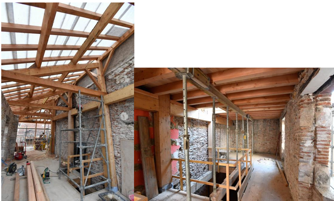
58 Figure A.2 - View of the building during refurbishment 59 60 61 62 63 64 65
