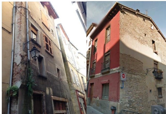
Figure 3: Cahors (left) and Vitoria-Gasteiz (right) demonstrator buildings
