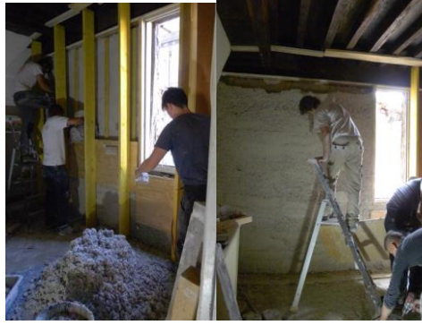
Figure 6: Refurbishment of an external wall with apprentice craftsmen, source [56]
