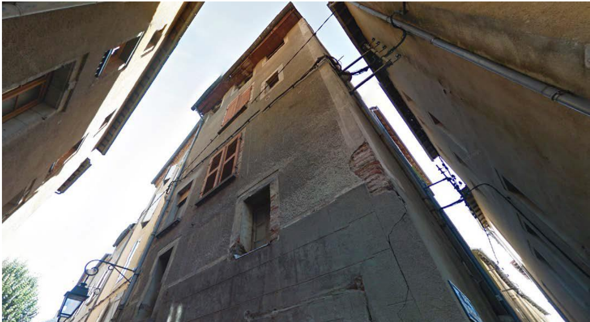
34 Figure A.1 – General view of the building before refurbishment 35
