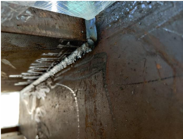
Figure 5-3 Welded joint between two main plates.
