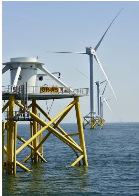
Figure 4-15 Close view of the jacket support structure of an OWT [119]
