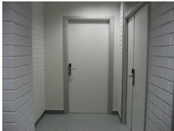
Figure 8.13: New doors at the Faculty of Computer Science
