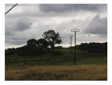
Figure 2. Medium voltage (MV) cables on poles.
