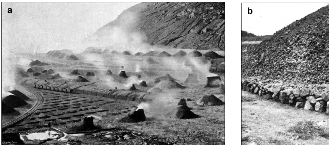
Figure 2.11. (a) Picture of open-air calcination of pyrite in Río Tinto mine (Nash, 1904); (b) base of a heap leaching (Pinedo Vara, 1963).
