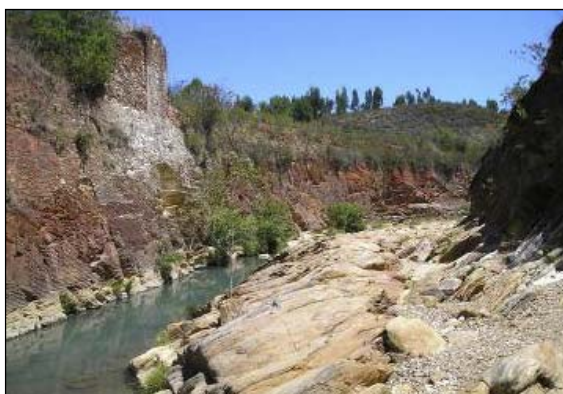
Figure 2.6. Retaining wall built for the diversion of Olivargas river, which natural course traversed the mine. Taken from López-Pamo et al (2009).
