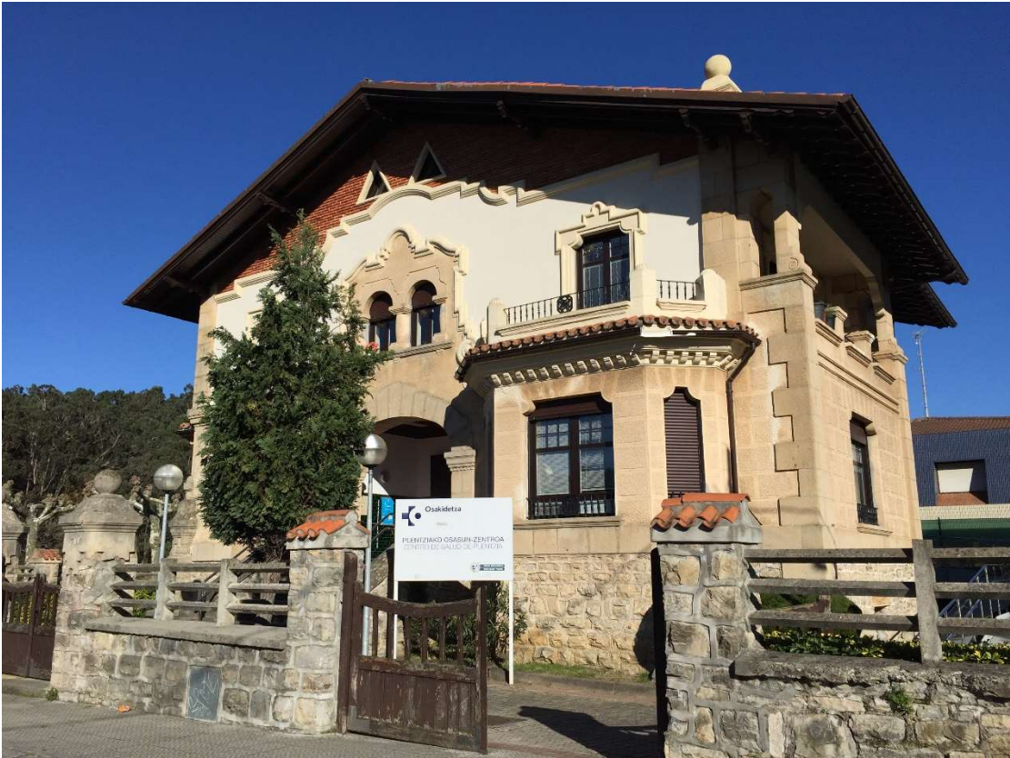
Figure 0.5. Local Health Centre at 4 Frontoi Street.
