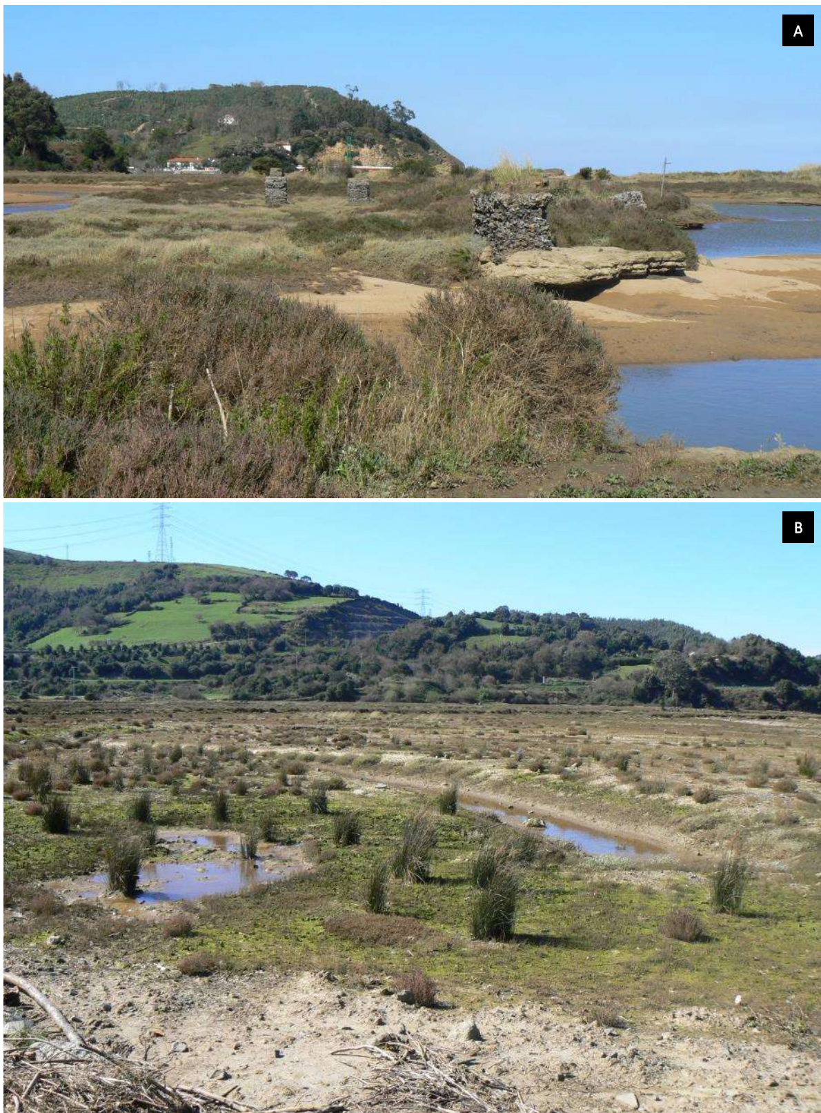
Figure 3.41. A. Barbadun salt marsh. Well preserved salt marsh vegetation can be seen and also several old industrial pillars, remnants of the mineral-ore transport activity to the loading bay in Covarón during the 19th century (Montero García, 1988). The buildings at the back are located in Pobeña, very close to the salt marsh of the same name. B. CLH marsh, with artificial gravel sediments, human-made channels and few planted reeds.
