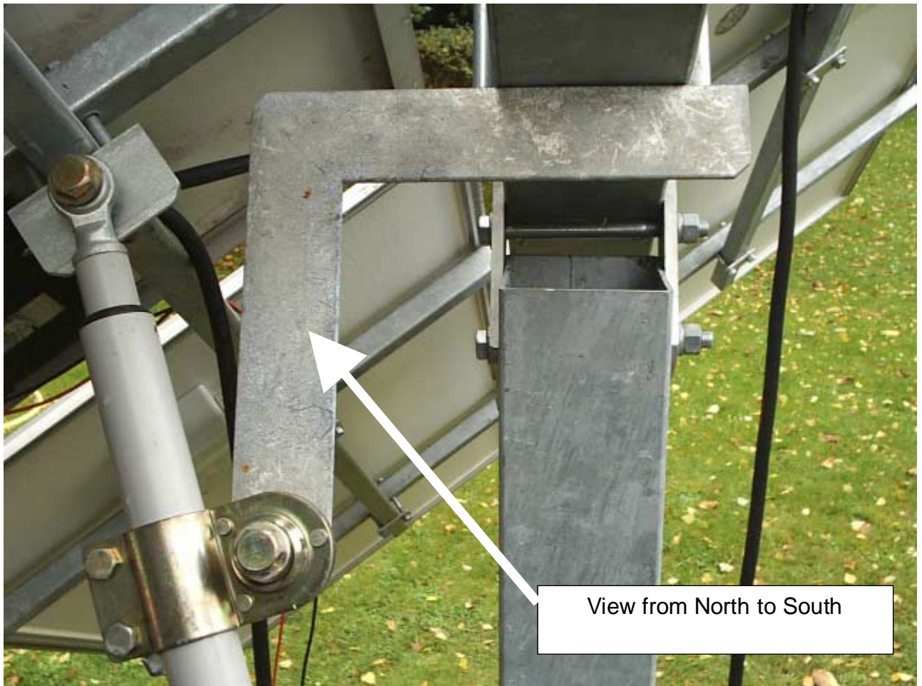
Lower Motor Fixation
