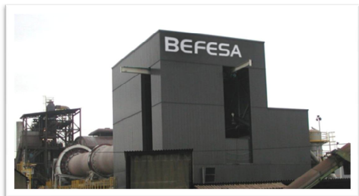
Planta Waelz – BEFESA ZINC ASER (by BEFESA)
