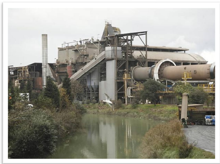
Planta Waelz – BEFESA ZINC ASER (by BEFESA)
