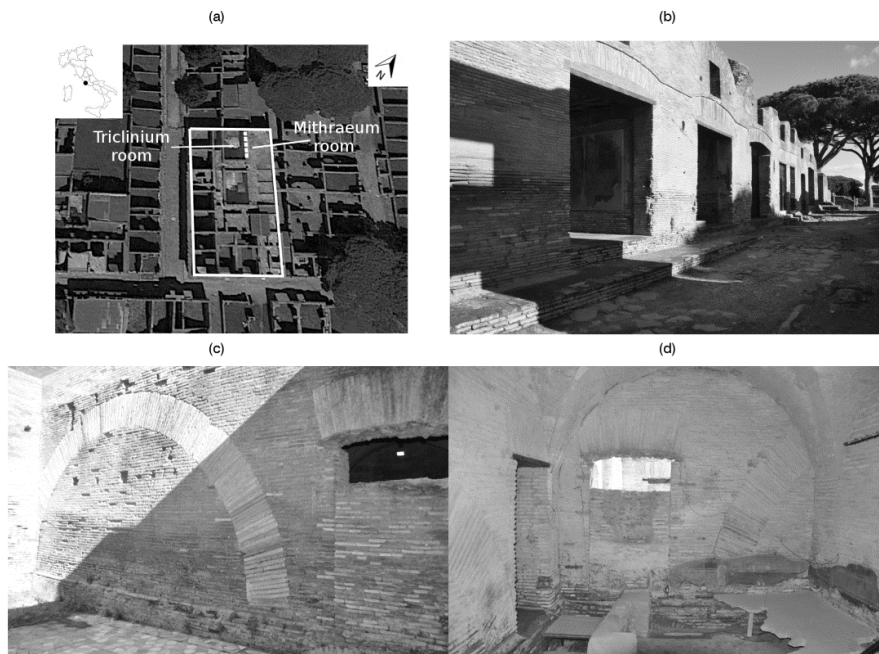
Figure 1. a) "Casa di Diana" at the Ostia Antica archaeological site (indicated with a white rectangle) and location of the "Triclinium" wall (dashed line); b) street view (Via di Diana), c) outer face of the "Triclinium" wall located in the Triclinium room; d) inner face of the "Triclinium" wall located in the Mithraeum room.
