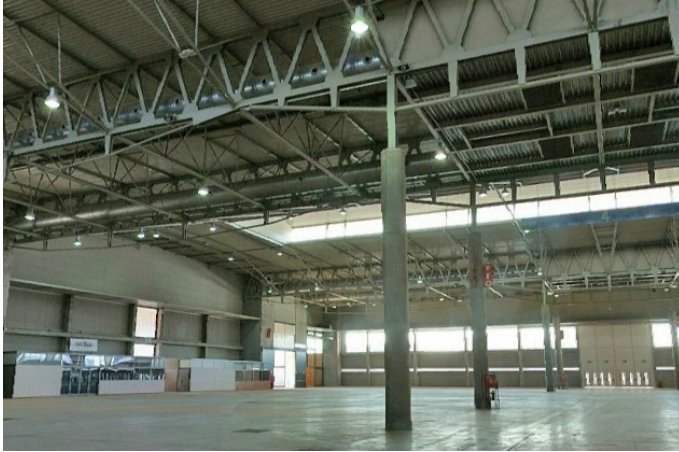
Figure 13. View inside the Barcelona Exhibition Centre building
