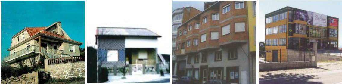
Figure 3 to 6. Common buildings normally considered 'ugly' in North Portugal and Galicia (Source: Villanova, Leite and Raposo 1995, 129; Lizancos 2000, 10; Paz 2006, 38; Domingues 2009, 244).
