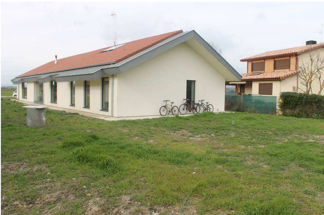
Figure I. 14. Monitored house view of the Southeast corner.
