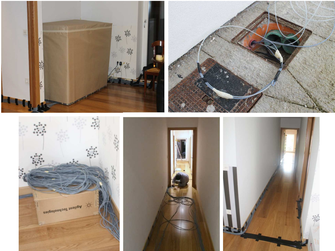
Figure 3.26. Acoustic box for datalogger and laptop (top left side), crossing cables to outside sensors (top right side), installation of cables and finished works on-site (bottom).
