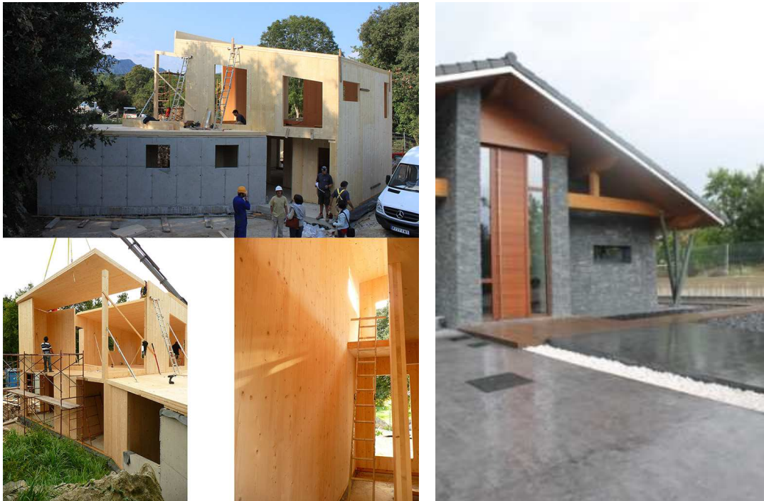
Figure 2.16. Examples of wooden structure in “casa entre encinas” (left side) and “Cagical Passivhaus” (right side) (data source: PEP & PHI, 2017).
