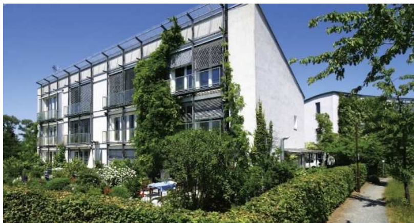
Figure 2.5. First Passive House in Darmstadt-Kranichstein (source www.passivehouseplus.ie )
