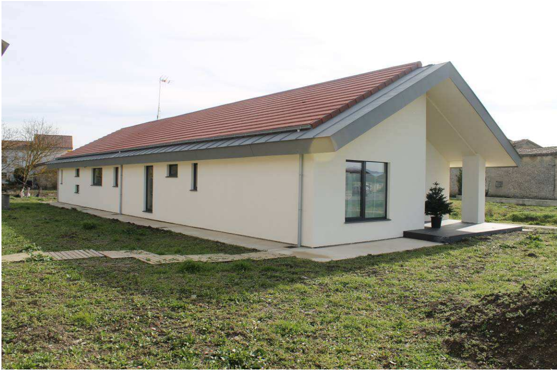
Figure I. 13. Monitored house view of the Northwest corner.
