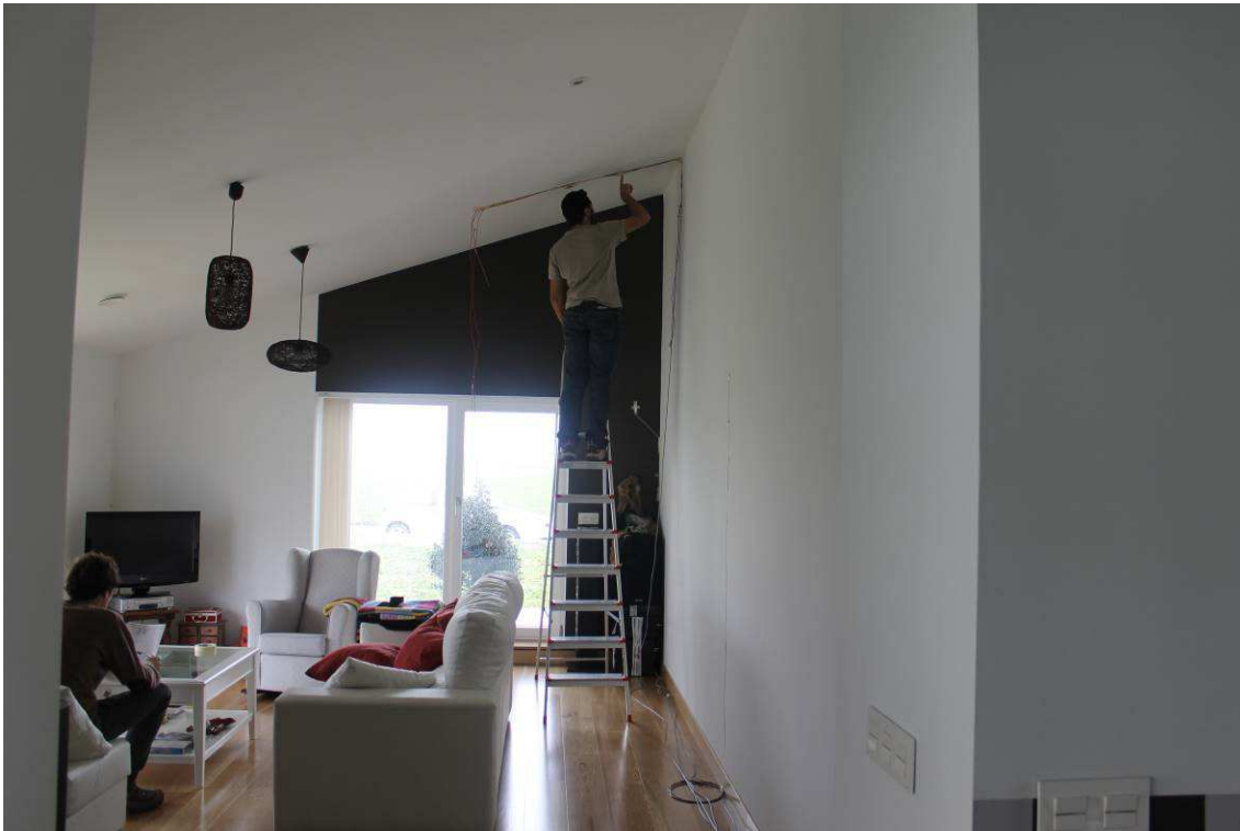
Figure I. 17. Details of the monitoring installation process, living room air sensors.
