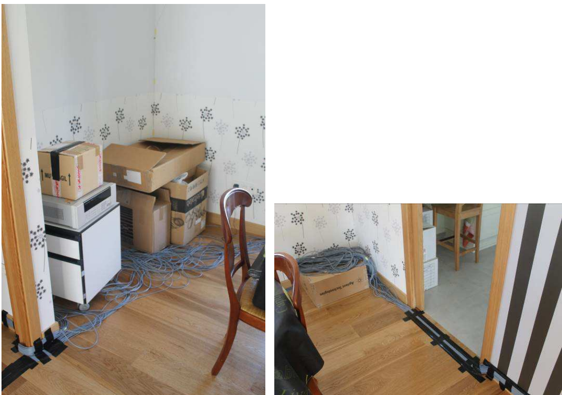
Figure I. 18. Details of the monitoring installation process.
